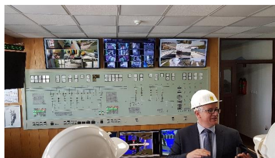
On the second day of the Seminar a study visit to HPP Čakovec was organized (pictured: a visit to the main Operating room)
